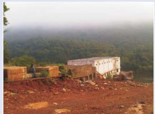
CAST STEEL SLUICE VALVE AT RISING MAIN OF A POWER PLANT
