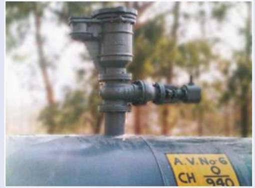
KINETIC AIR VALVE WITH ISOLATING SV
