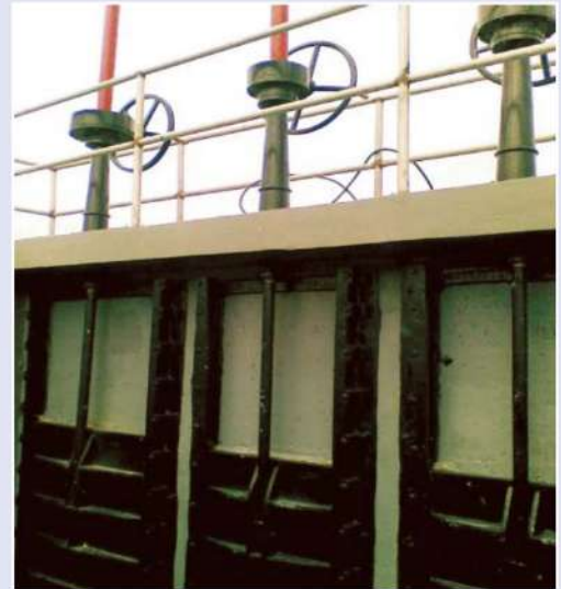
CAST IRON WALL MOUNTED SLUICE GATE
