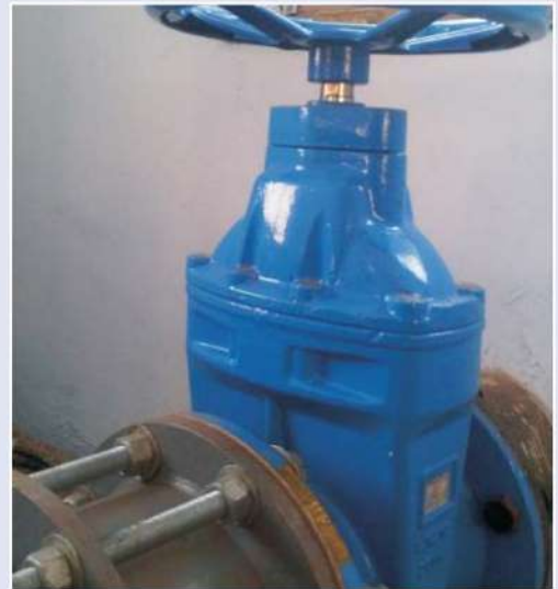
DI RESILIENT SEATED GATE VALVE
