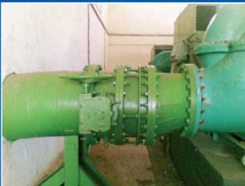
BUTTERFLY VALVE & DUAL PLATE CHECK VALVE
