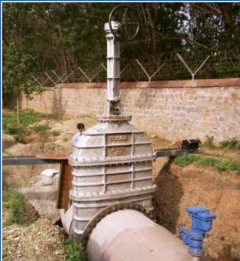
1500 MM CAST STEEL GATE VALVE
