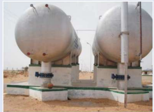
BUTTERFLY VALVES INSTALLED AT SURGE VESSEL
