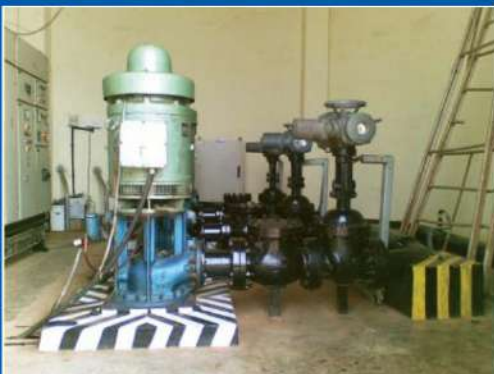
CAST STEEL CLASS 300 MOTORIZED GATE VALVES
